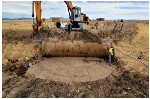
Hwy. 21, North of Sanford. We installed a new culvert and plans are to re-pave this road and install guard rails.
