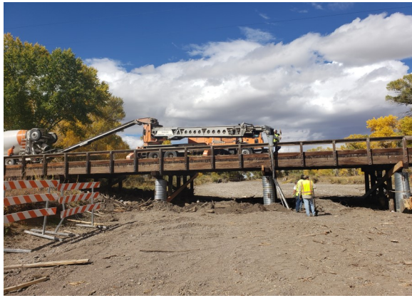
The bridge with the cement pumper truck is on county road V . The wood plank bridge is on county road 11 just north of county road H.
