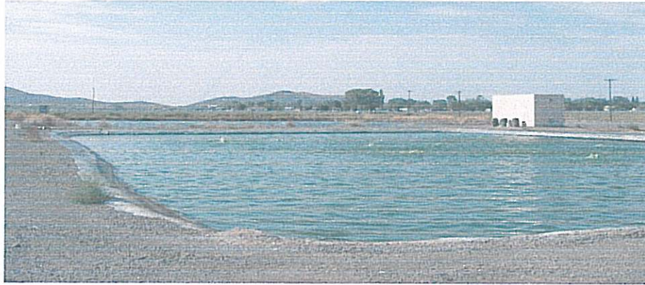
Figure 61 Waste Water Treatment Plant at Manassa
