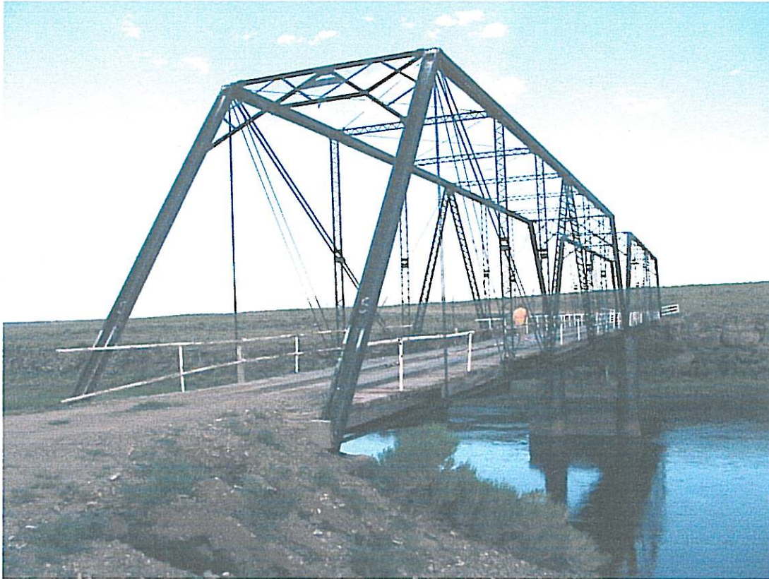
Figure 73 Costilla Crossing Bridge, AKA Lobatos Bridge
