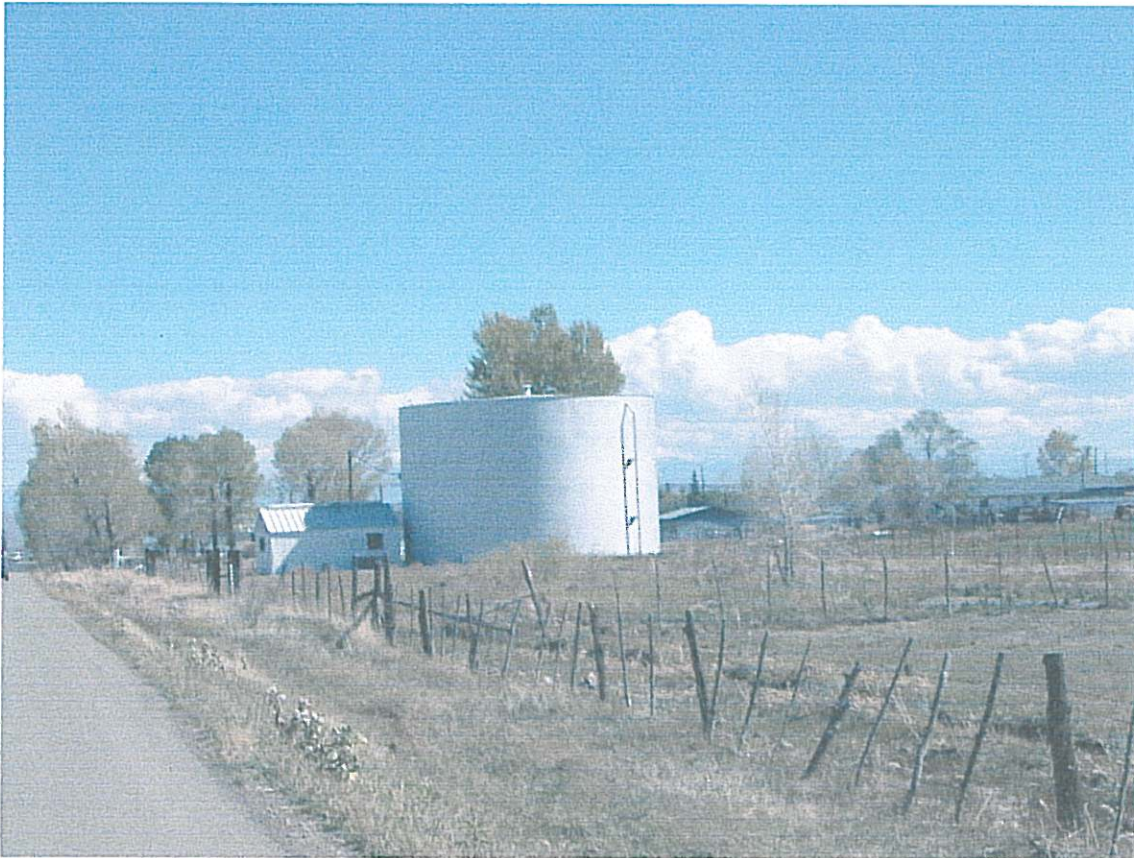
Figure 69 Antonito Water Distribution Site
